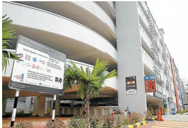
Figure 4. Park & Ride Gombak Station Malaysia
